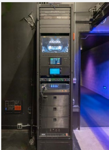
Backstage, PCD installed video monitors and speakers, as well as paging system so the actors can hear their cues.
